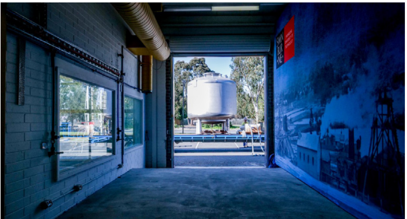
SABRE South vessel delivered at SUT (Wantirna site)
